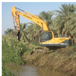
Maintenance of irrigation channel with heavy machinery
