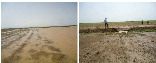
Jidah made to collect water and a ridge partly damaged by a strong water flow
