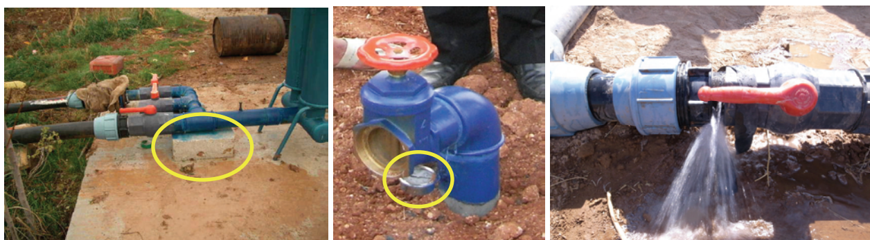
Left: Use of a brick instead of a pedestal makes durability problematic.
