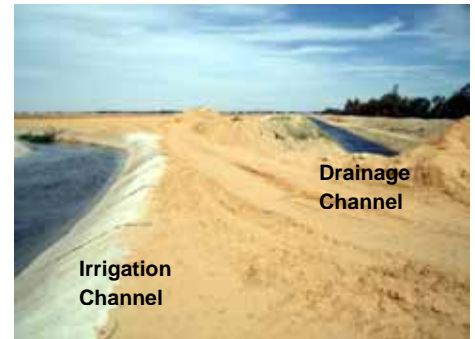
Irrigation channel and drainage in newly opened farm land
