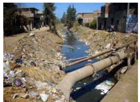
A drainage channel in the Nile Delta
