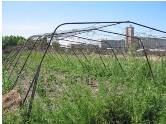
Derelict iron piped greenhouse
