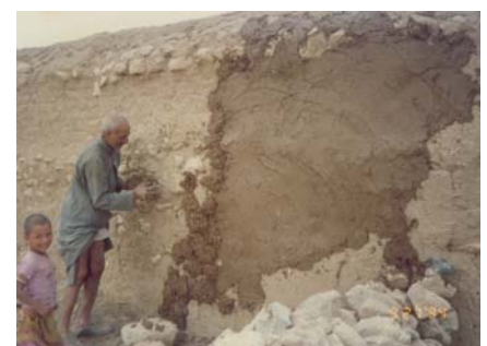
Renovation of sun-dried brick house
