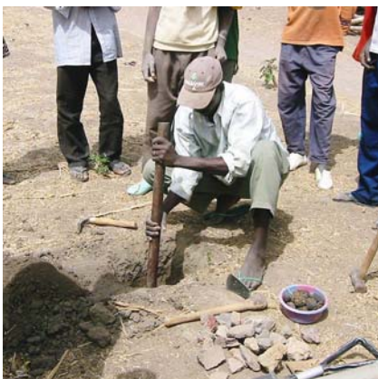
Digging a pit using locally available tools
