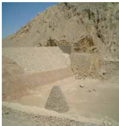
Construction of a delay action dam
