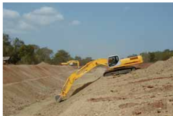
Construction of canal (main 19km, tributaries 24km)
