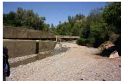
Intake weir in use for several decades
