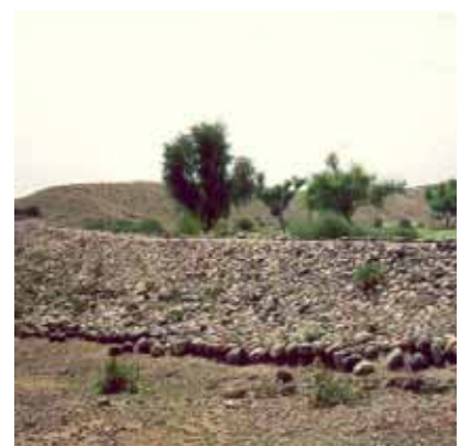
Dam for water-harvesting (Pakistan)
