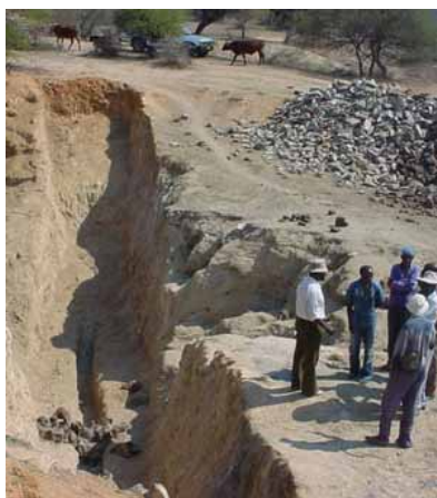
Small-scale dam maintenance work
