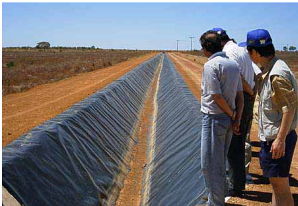
Irrigation channel construction (Brazil)
