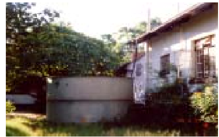
Photo 2: Water tank made of galvanized iron sheet
