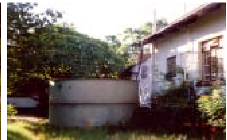
Photo 2: Water tank made of galvanized iron sheet
