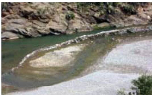
Small-scale water weir built by a traditional method
