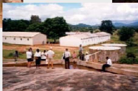
Rainwater collection facility using the rock surface (with a primary school building in the background)
