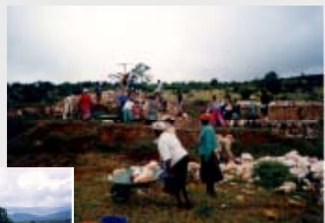
Constructing a dam by local people
