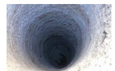
Underground pits for wastewater, digging to reach the water level
